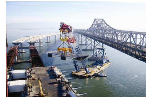
Working site for erection of New Bay Bridge with crane vessels provided by ZPMC
