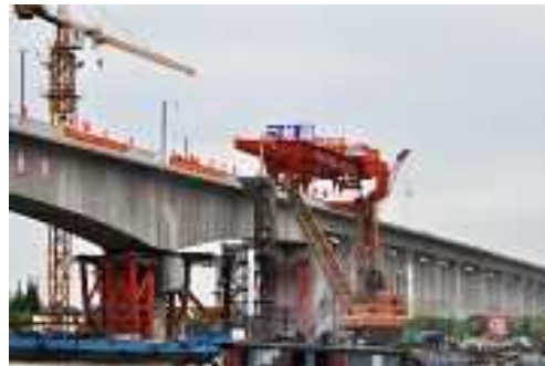
Completion of Girder Erection project for Shanghai-Hangzhou PDL
