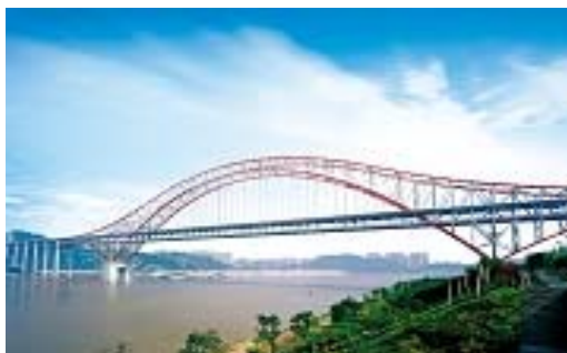
Chaotianmen Yangtze River Bridge, with the longest span of steel-box girder globally
