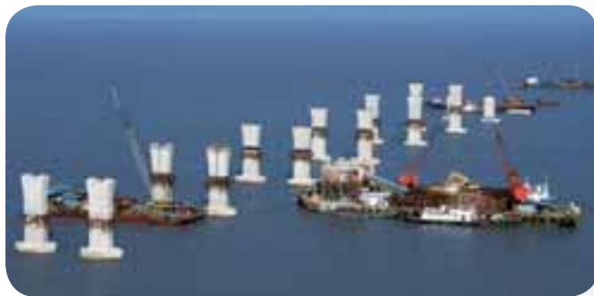
Installation of precast tower pillars
