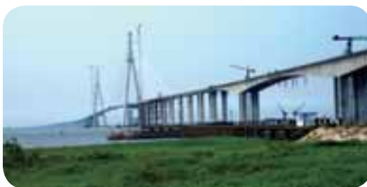
Sutong Bridge upon closing
