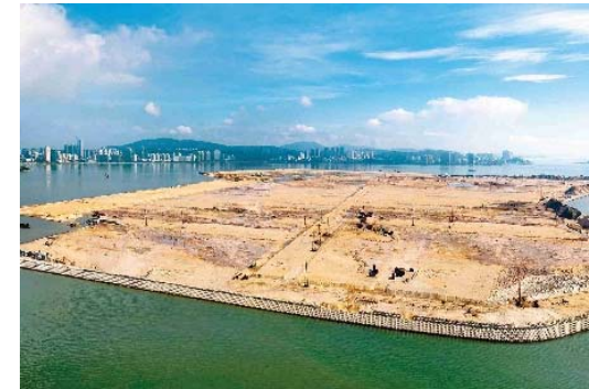
Reclamation dredging for West artificial island of Hong Kong-Zhuhai-Macau Bridge
