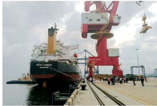
Kribi deepwater harbor in Cameroon
