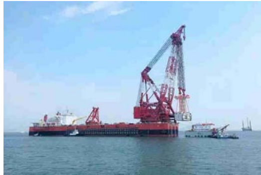
12000t self-propelled revolving floating crane is on work
