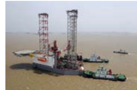
The first Drilling platform constructed by ZPMC successfully launched
