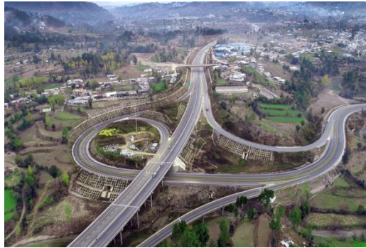
Full Opening of Karakoram Highway Phase II
